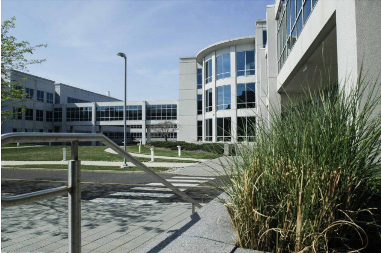
The New Jersey Center of Excellence in Bridgewater — Courtesy: Advance Realty
